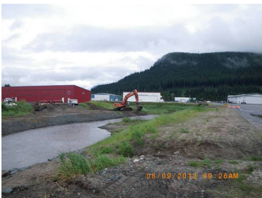
This image, taken on August 9, shows bank restoration efforts at Jordan Creek, just north of Taxiway A.
