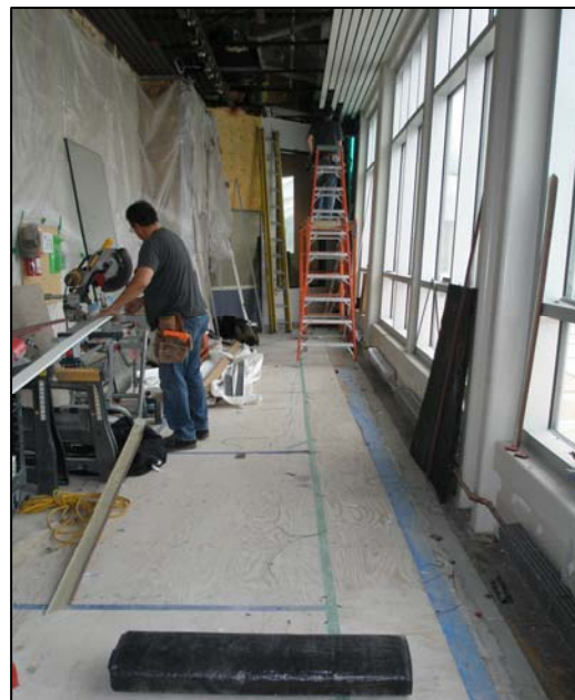
Ceiling installation underway in restaurant.
