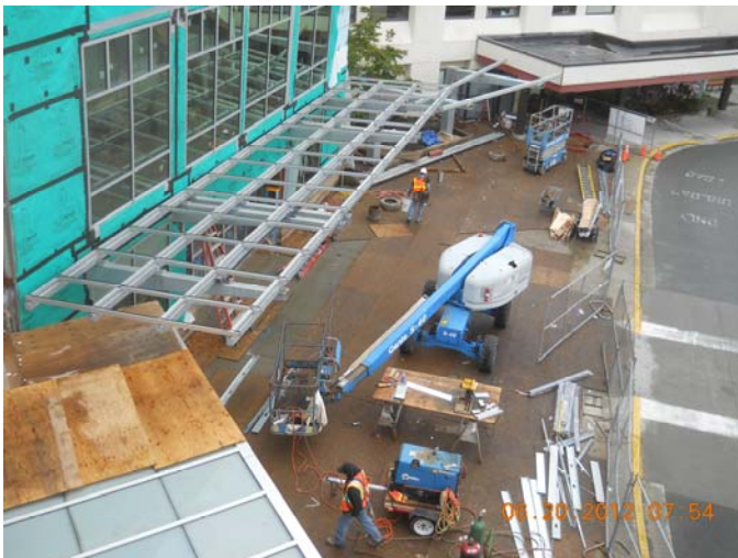
Canopy framing installed at main entry.
