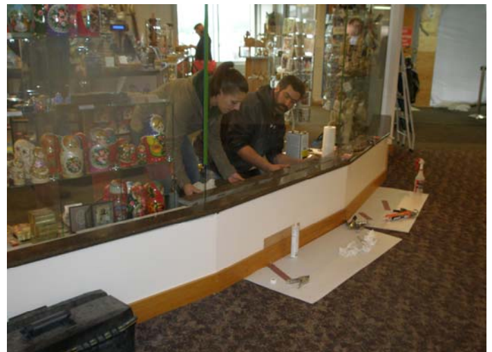
Quartz sill is installed at Hummingbird Hollow gift shop.
