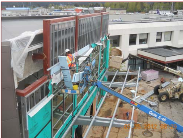
Welding at front entry.
