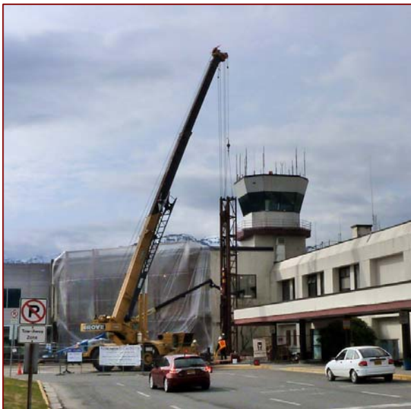
Pile driving for new canopy columns.
