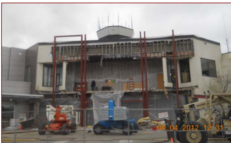
Primary steel is installed on the front facade.
