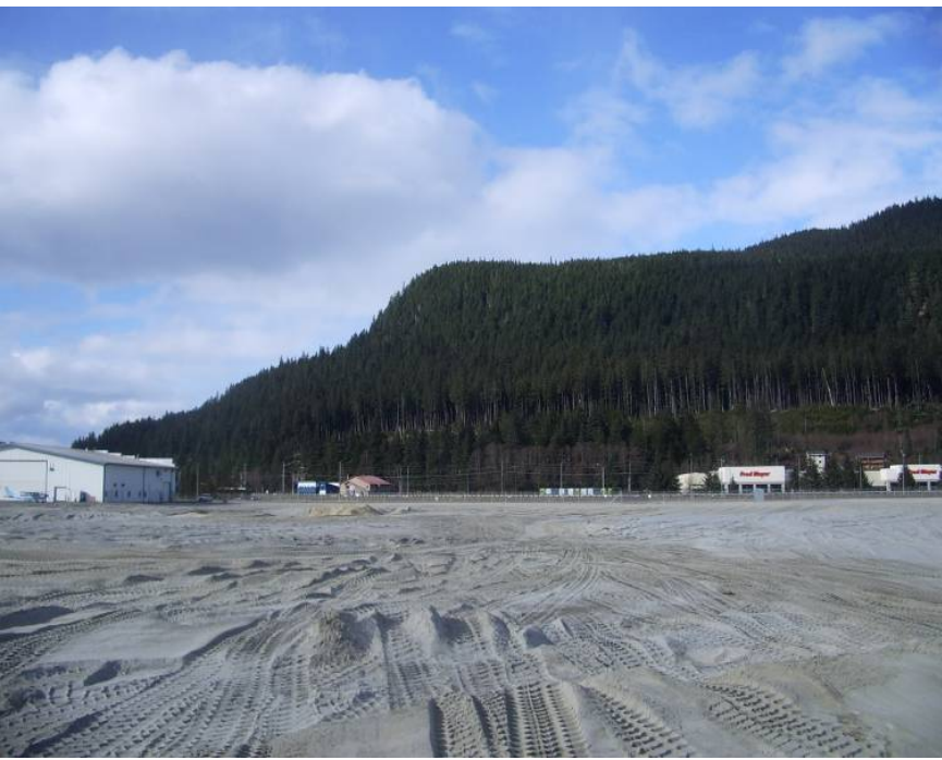
This March 31 image was taken from the edge of Taxiway A looking north across the N.E. Development Area. The Wings of Alaska hangar is visible to left, Fred Meyer is visible in the distance to the right. All stockpiled material has been placed and final grading is underway.
