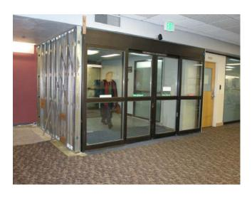
Depth of entry vestibules in the terminal's North Wing are increased to minimize heat loss.
