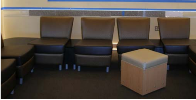
Chair rail trim made of leftover terrazzo tile will prevent damage to wall surface in Departure Lounge.
