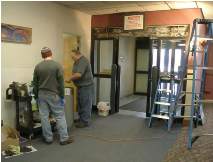
Door Repairs at Gate 1, North Wing.
