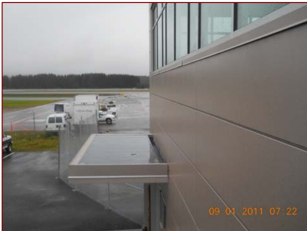
Punch list completion includes repair to roof canopy and revising cowling flashings to stop water leaks.
