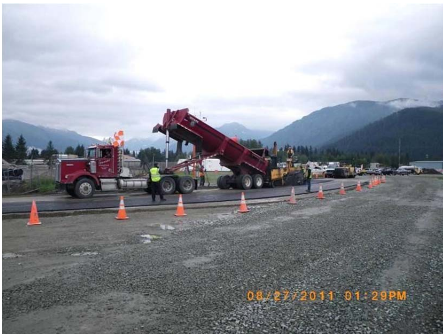
Paving float plane access road.
