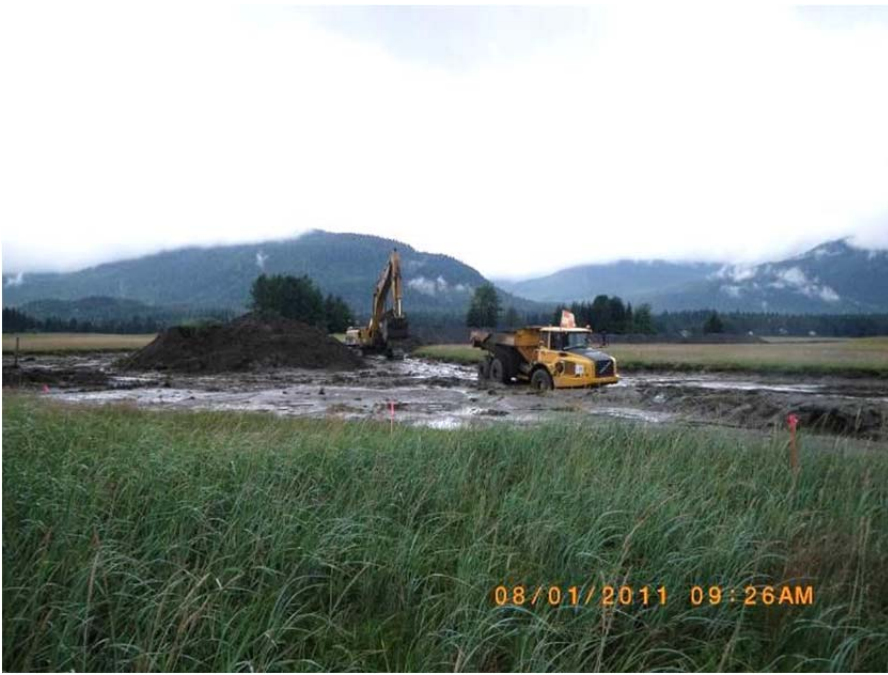
Excavation of organic overburden from relocated East Runway Slough.
