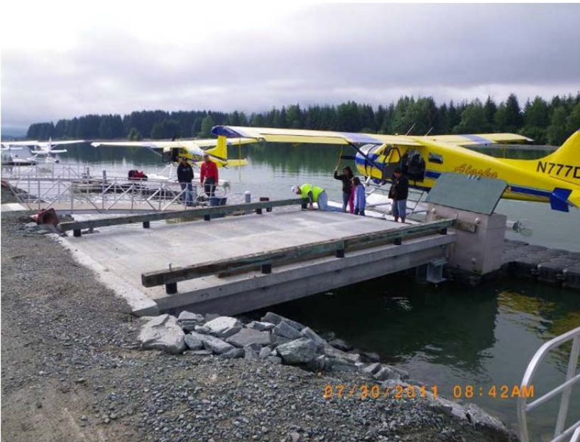
20 foot loading platform with bull rails at Alaska Seaplanes.
