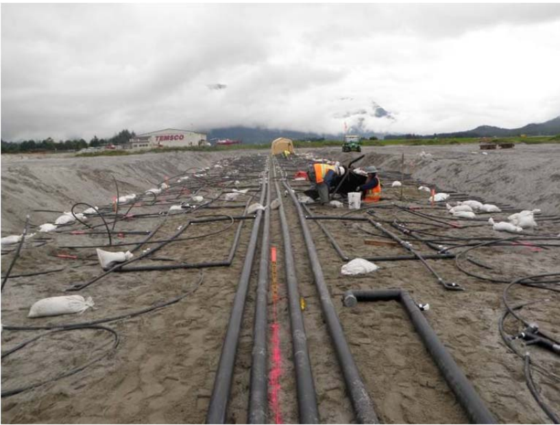
Loop field manifold installation.
