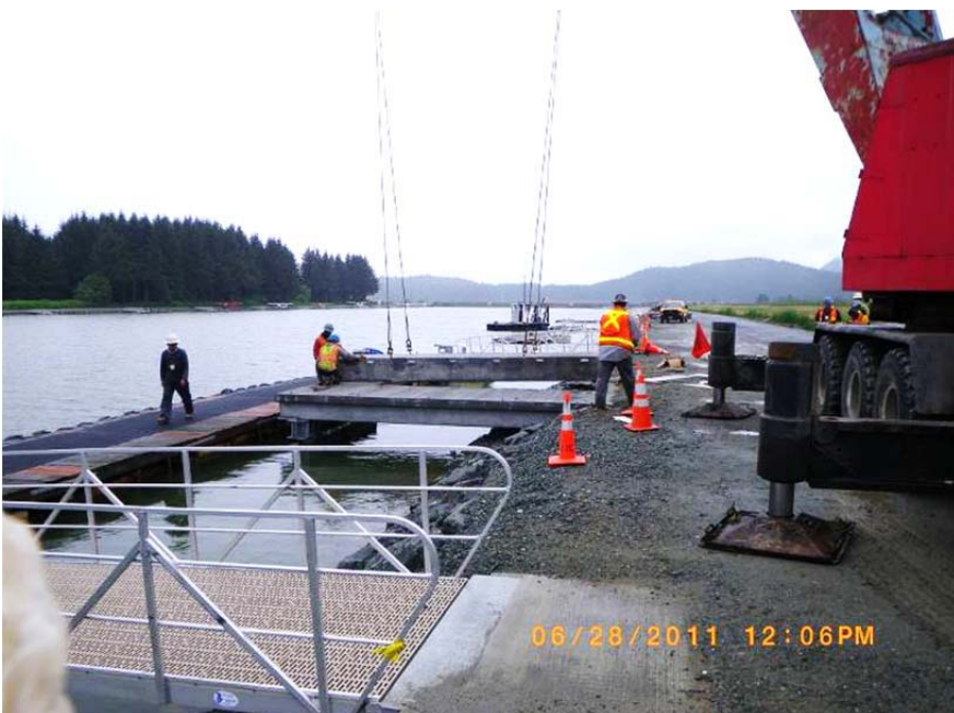
Initial placement of concrete loading platforms
