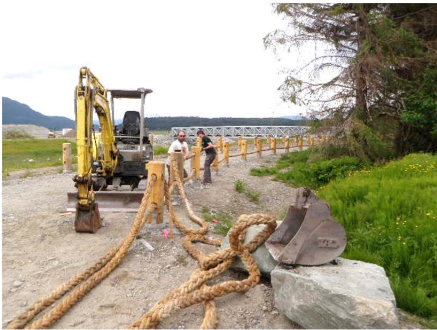
Pulling rope for the Log Post and Rope Fence.
