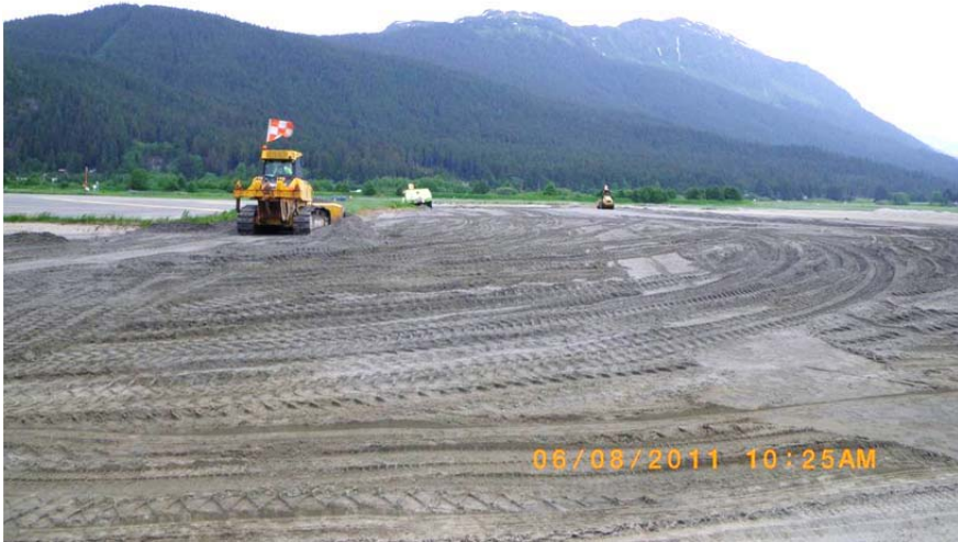
Placing material from East Finger at East RSA
