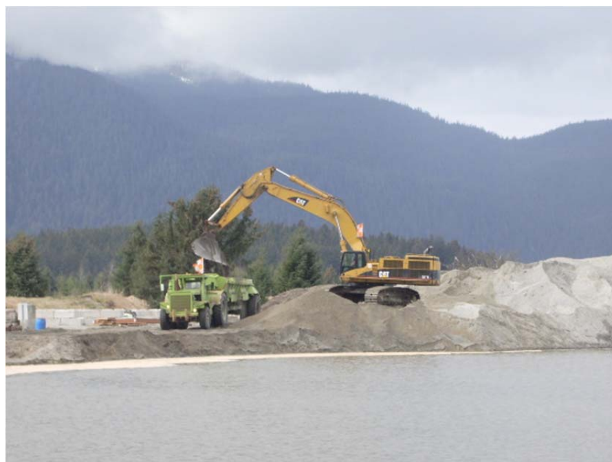
Truck haul of stockpiled material from south shore of pond.
