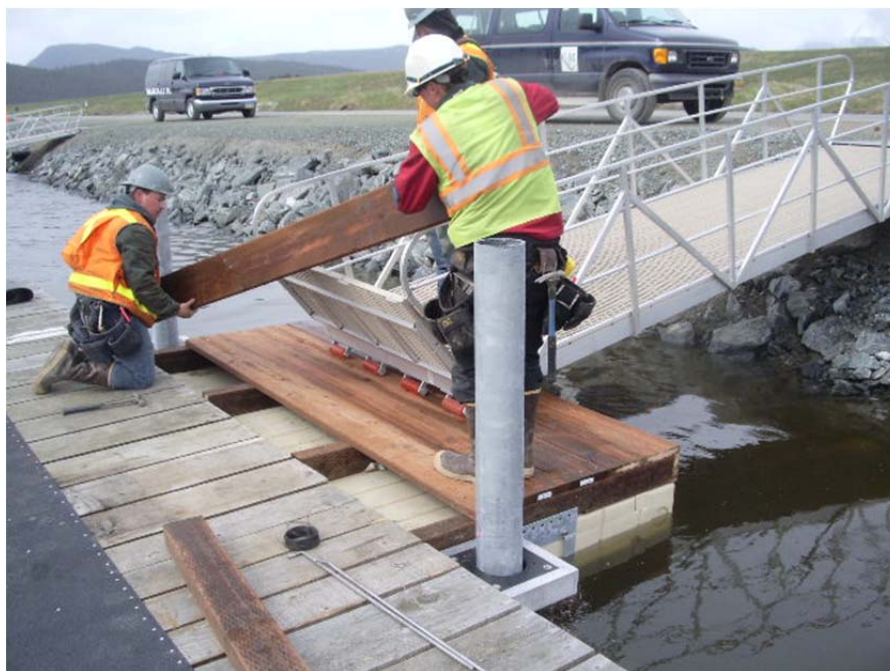
Detail work to mate an EZ Dock to an existing float.
