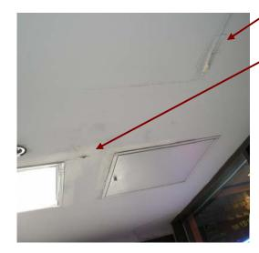
Main entry vestibule ceiling damage from frozen sprinkler line located in ceiling.
