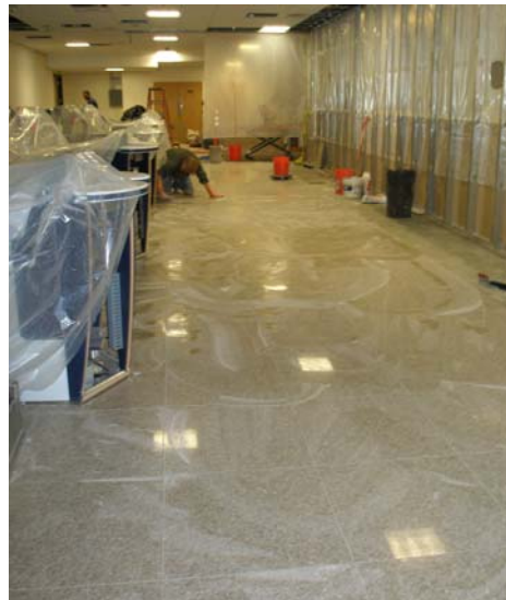
Grout installation at Check-In lobby.
