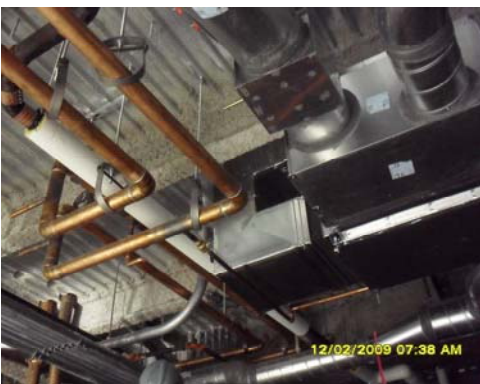
A total of 26 Water-to-Air Heat Pumps are installed in ceiling spaces inside the building.
