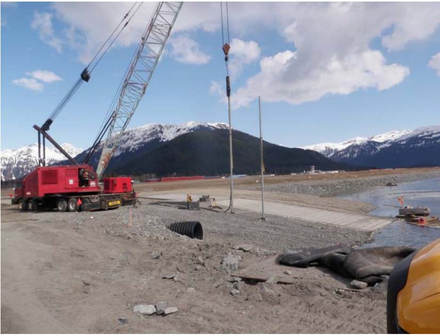
Northwest launch ramp - piles driven for new dock
