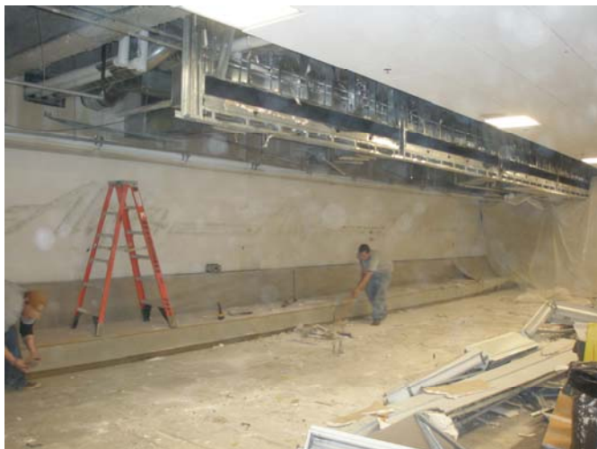
Demolition at Check-In Lobby.
