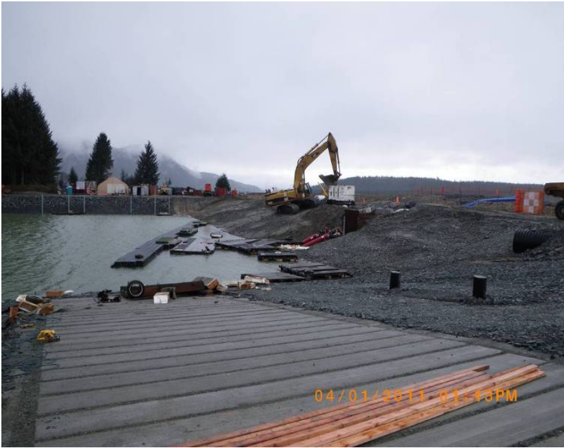
Northwest launch ramp nears completion
