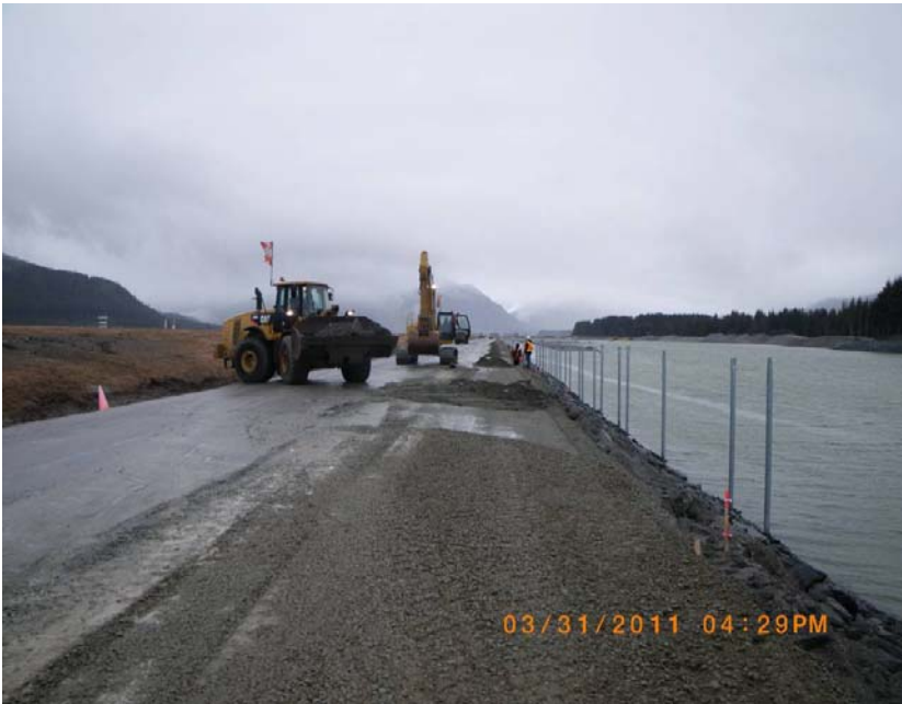
Placing D-1 shoulder on north shore
