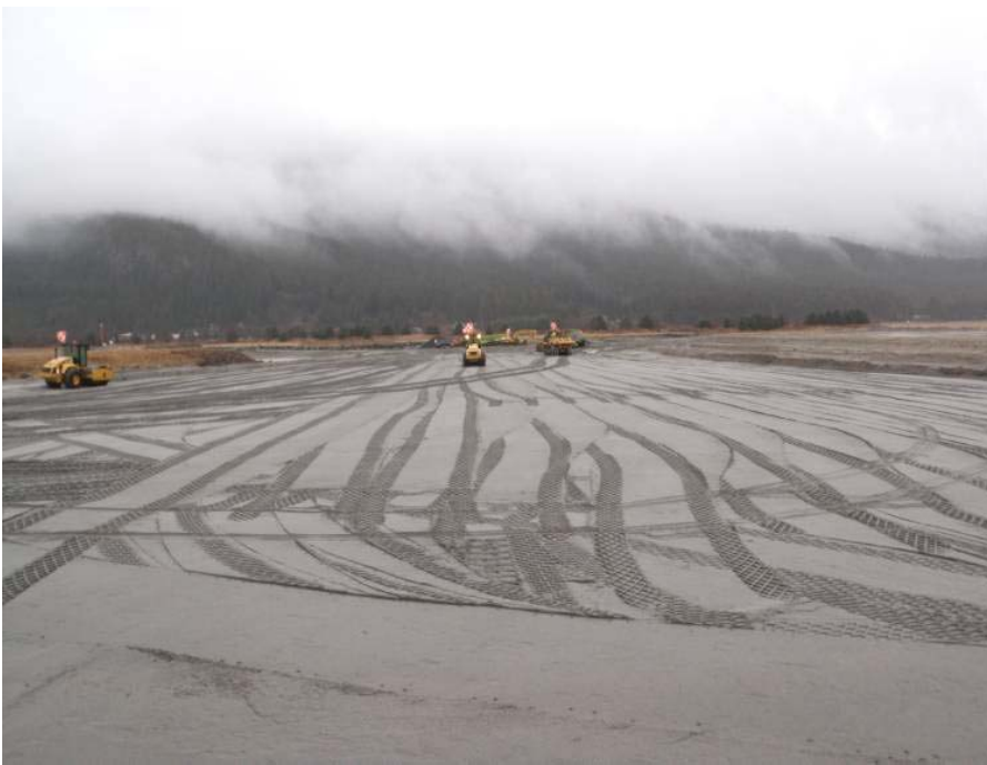
Compacting embankment at East RSA
