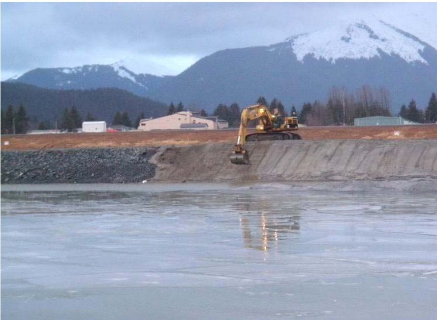
Shaping the north shore side- slopes
