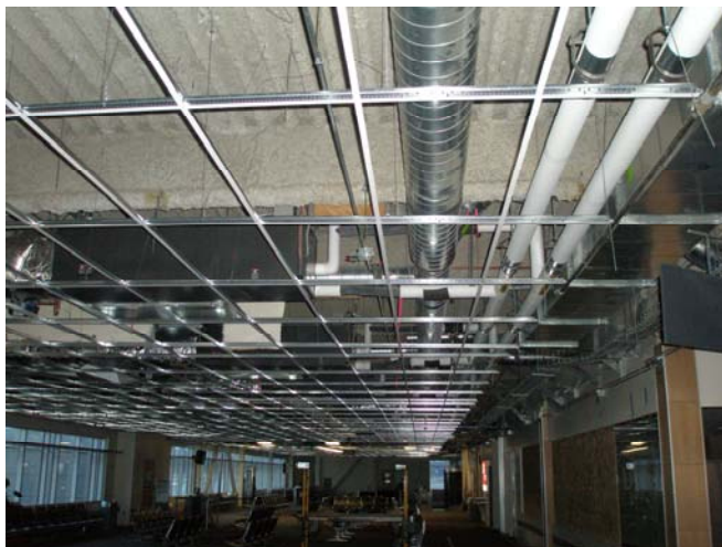
Install of ceiling grid in Departure Lounge
