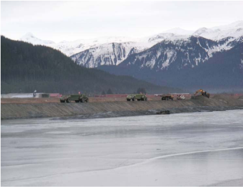
Excavation and haul along north shore of pond.
