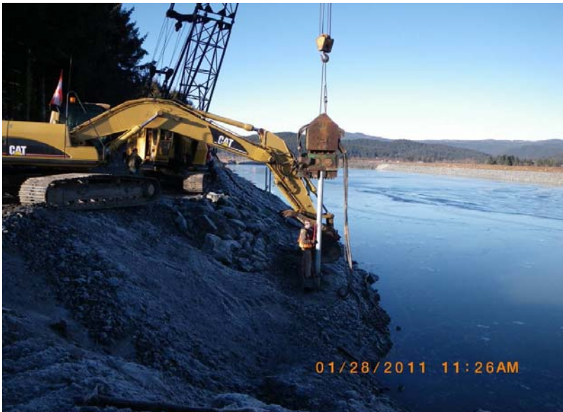
Driving 6" galvanized piles along southwest shore of pond.
