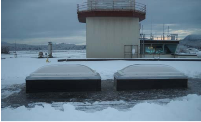
New skylights were installed over former mechanical shafts.
