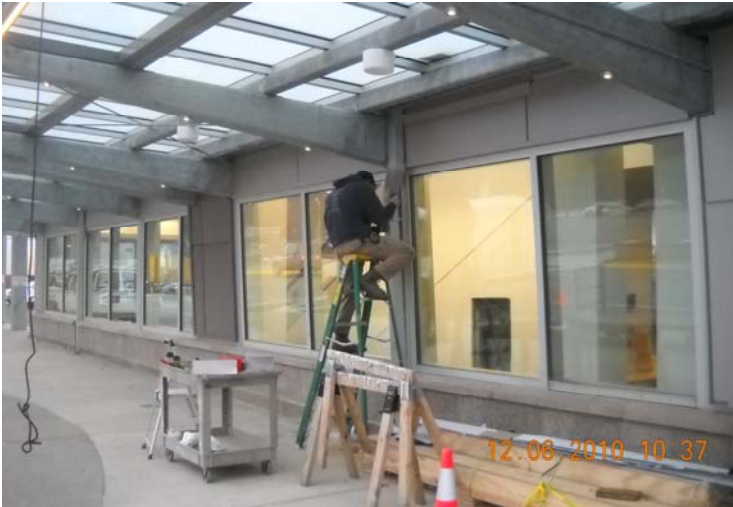
Exterior trim was completed during December, 2010.
