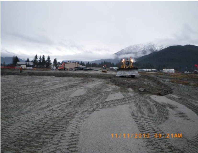
Placement of trucked borrow at West RSA.
