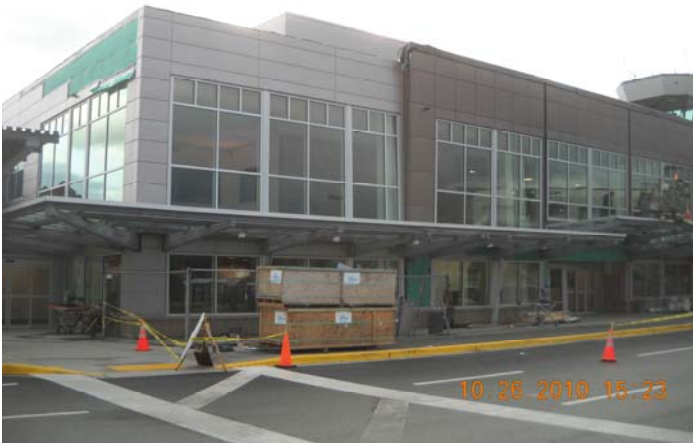
Siding at East end nears completion.
