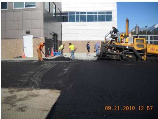
Paving at new tug entrance, East end.
