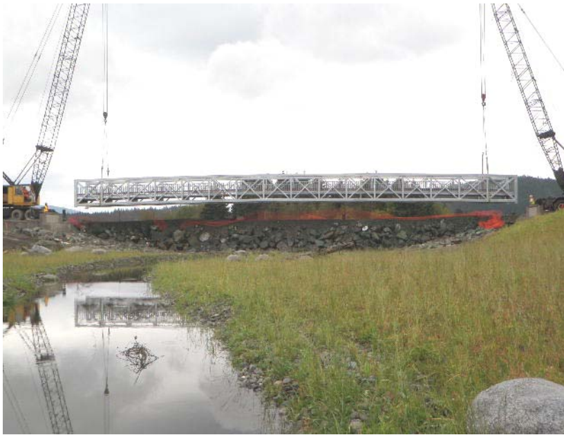
Placement of Duck Creek Bridge
