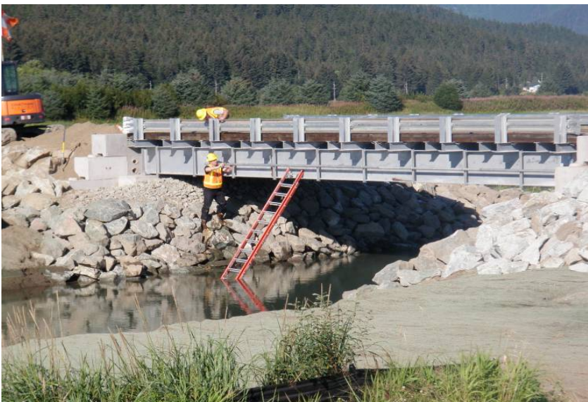
Bridge for new ASOS pad.
