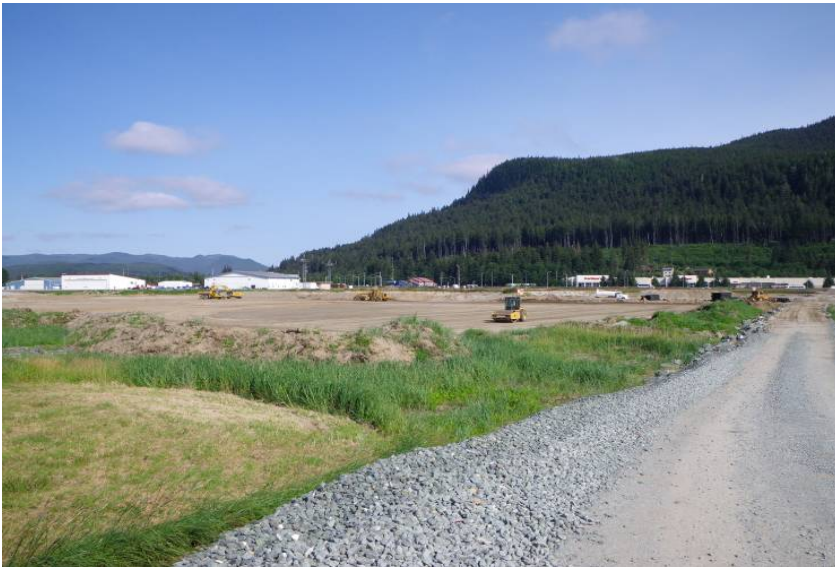
Grading for geothermal ground source loop field site.
