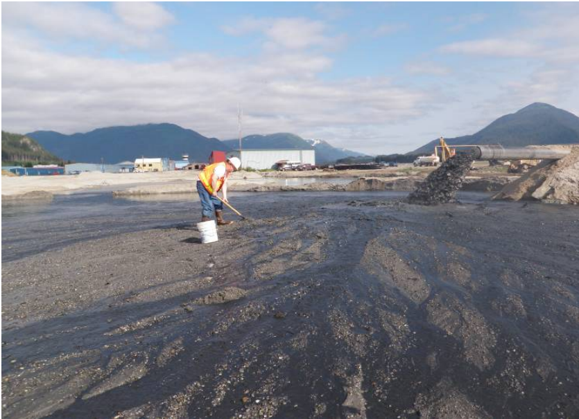
Placement of dredge material in Northwest Development Area.
