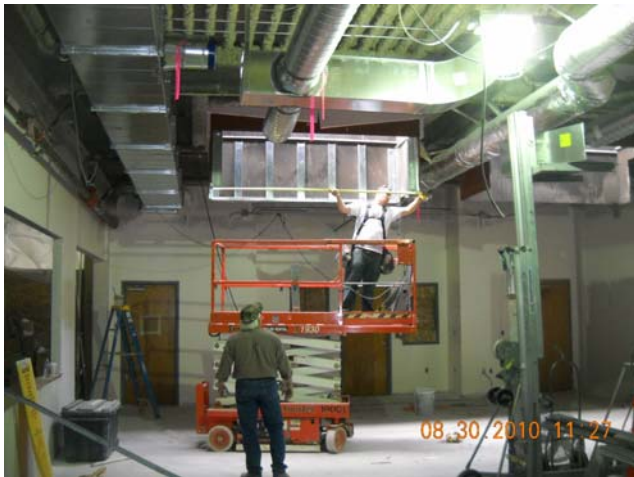
Reuse of mechanical shaft to new skylight in TSA Screening
