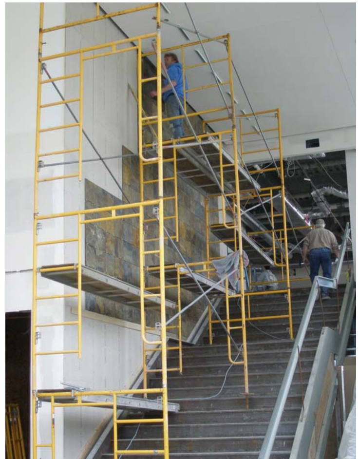
Slate tile installation near escalator.
