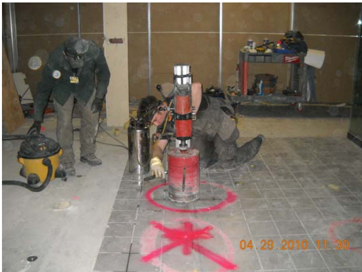
Core drilling for new plumbing lines.
