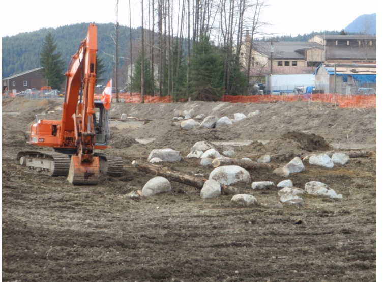
Duck Creek details underway
