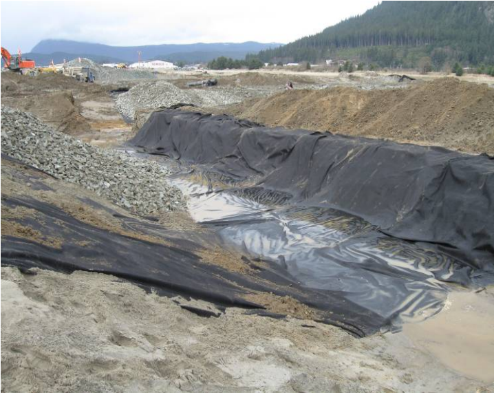
East end RSA rip-rap perimeter
