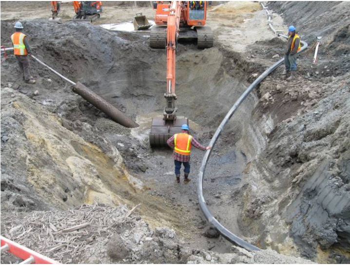
Bayview force main being lowered
