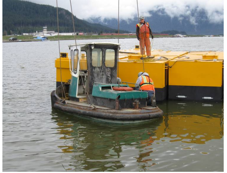
Dredge barge being assembled
