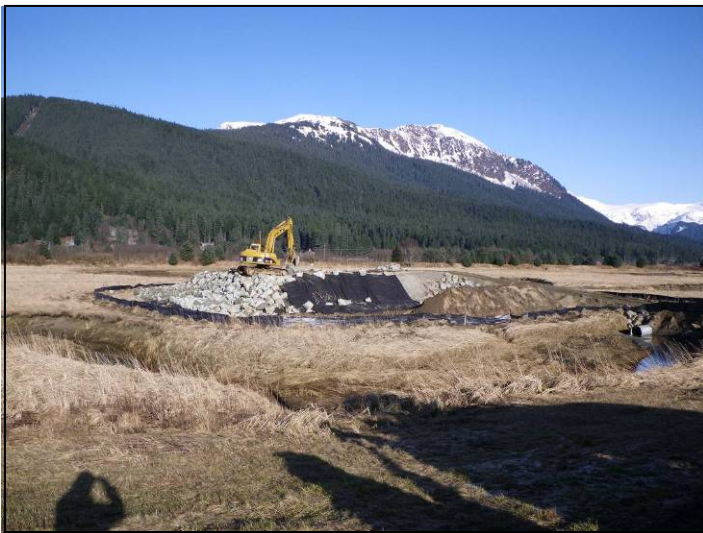
Placement of rip-rap slope protection for ASOS Pad.
