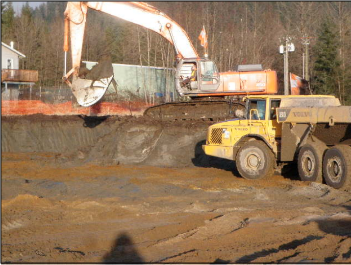
Excavation of unsuitable material at Duck Creek
