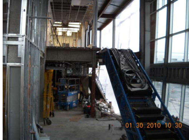
The new escalator is in place
