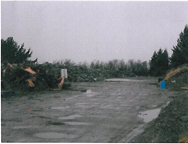
Class B underlayer rock at east end of pond
