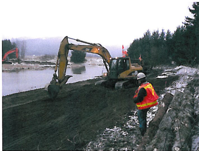
Clearing & grubbing on west finger road alignment
