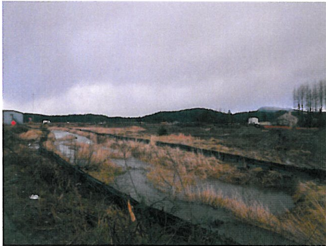
Silt fences, clearing on Duck Creek
