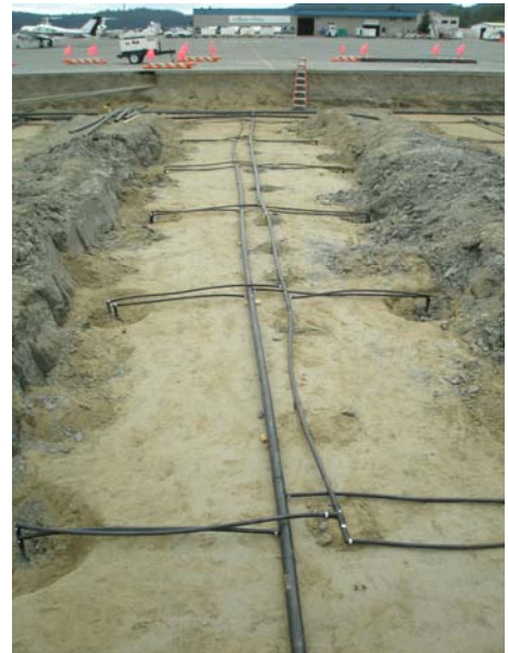
7.15.09: Manifold in trench is complete.
