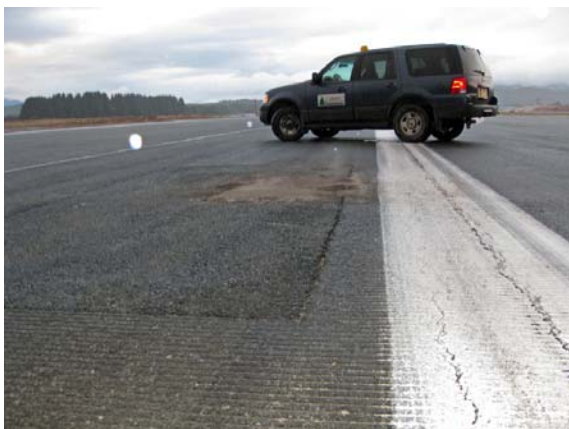
Finished interim repair
