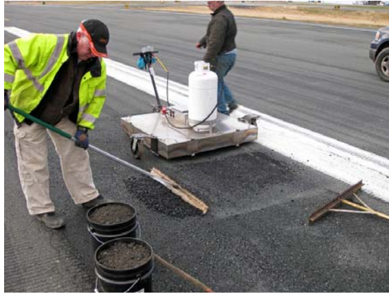
After heating, work the material
