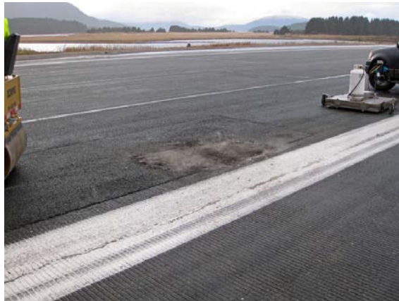
Finished repair (more to come...)
