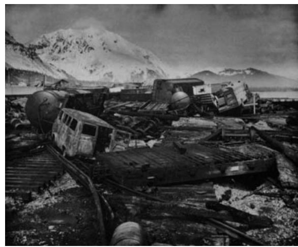
Tsunami damage at Seward, Alaska
