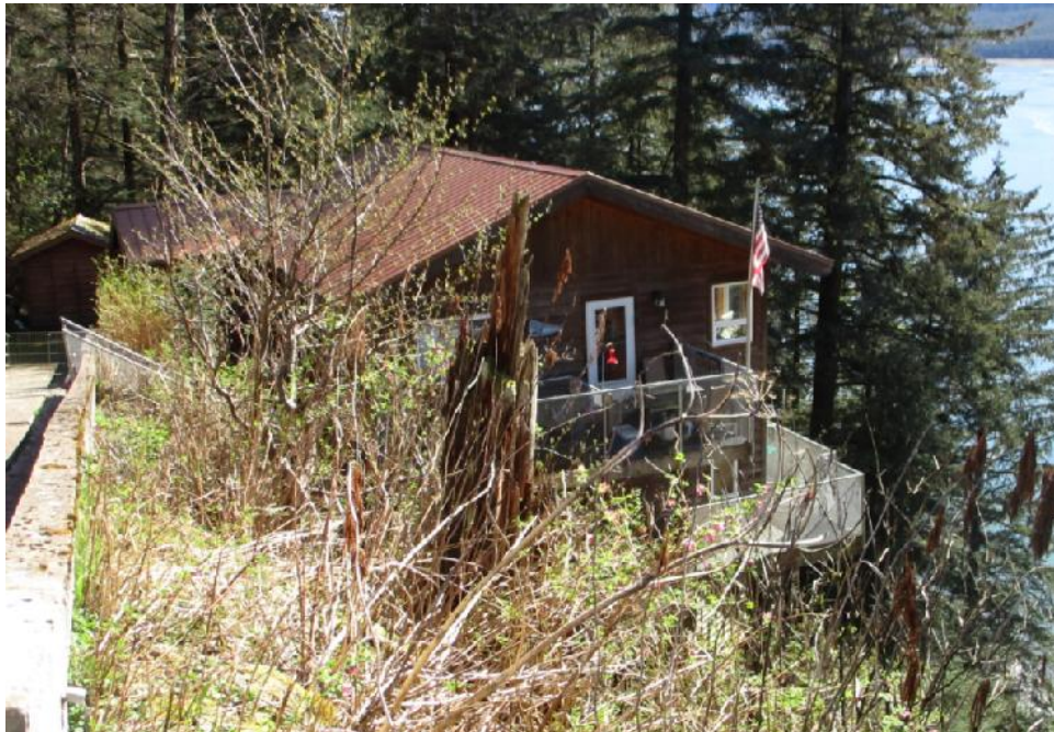
Residence North Side View
