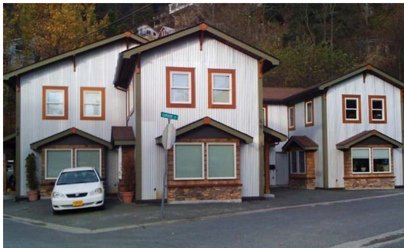
Attention to Scale and Context Attractive new 4-plex along Village Street with durable and stylish metal siding.
