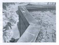
Other similar buildings have experienced significant damage due to bird activities on both horizontal and vertical EPDM membranes to the point that the roof had to be replaced.
