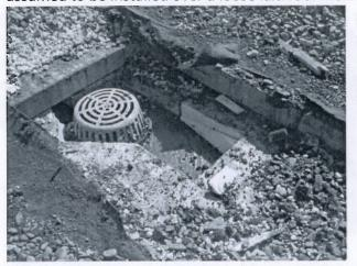
gypsum sheathing where the roof deck is installed over steel deck. It is assumed that the gypsum sheathing is omitted at the concrete slabs. Because the roof is installed in an inverted roof membrane (IRMA) configuration, there is no vapor barrier. Channels are provided in the roof insulation to promote drainage to the existing roof drains. The entire roof perimeter is lined with 6
