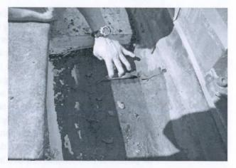
the EPDM base flashing to the asphalt membrane is an unusual condition requiring intermediate materials which likewise can be breaking down.
