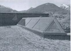
of the skylite includes a counterflashing similar to a Fry "Springlok" type counterflashing so that the membrane roofing can be removed without disturbing the skylite frame.
