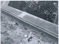
deteriorated, but the factory finish is beyond its useful life. The fasteners are likewise disintegrating.
