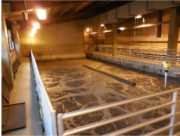
Figure 8. SBR in the Aeration (React) Cycle
