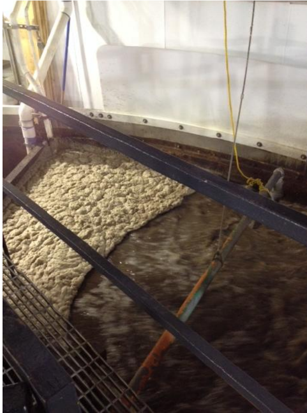
Figure 4. ABTP Contact Aeration Zone
