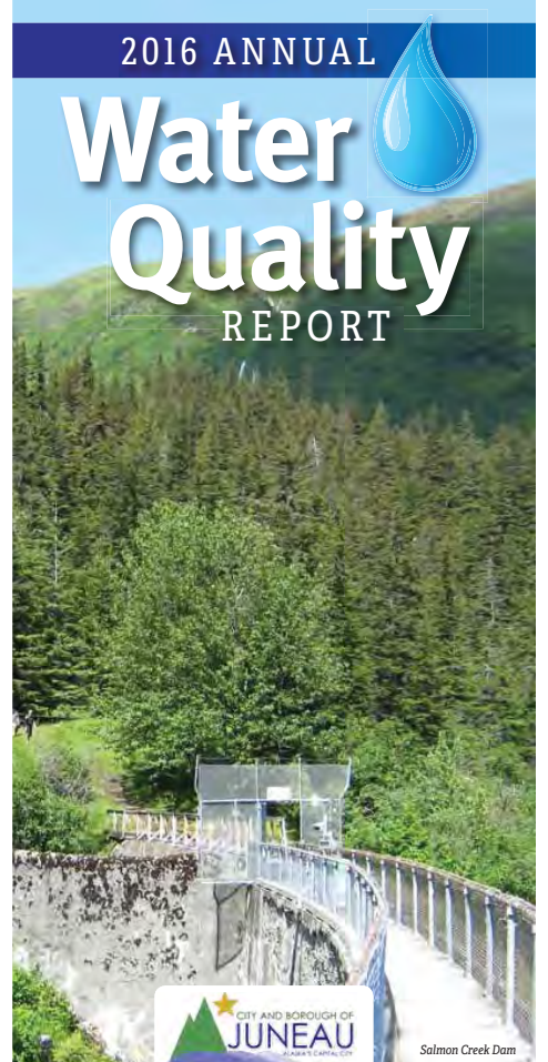
Salmon Creek Dam
