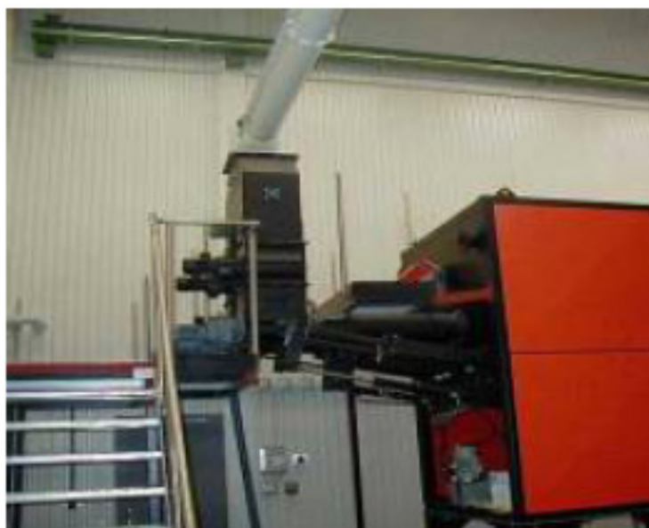
FIGURE 4 BioCon-ERS Incinerator Furnace
