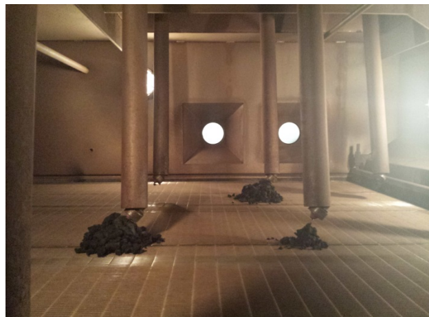
Figure 4. Sludge deposited on dryer belt by extruders
