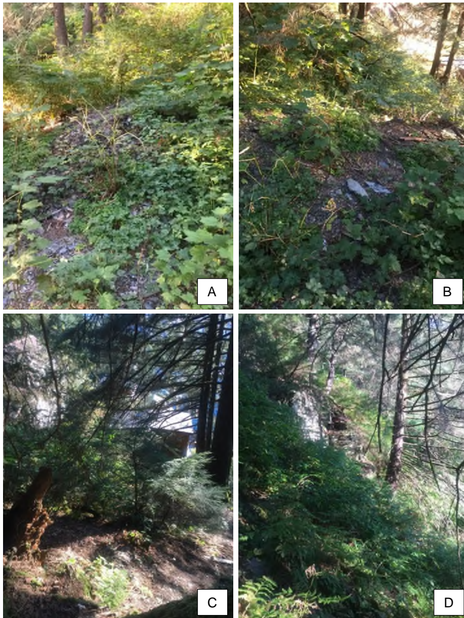
Figure 9: Active debris slide paths above Nelson Street are shown in Figures 9A and 9B; rock bluffs and broken or damaged trees above Nelson Street are shown in Figures 9C and 9D.
