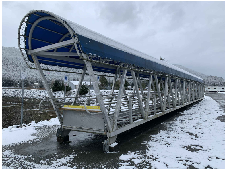
SALVAGED GANGWAY - NORTH VIEW
