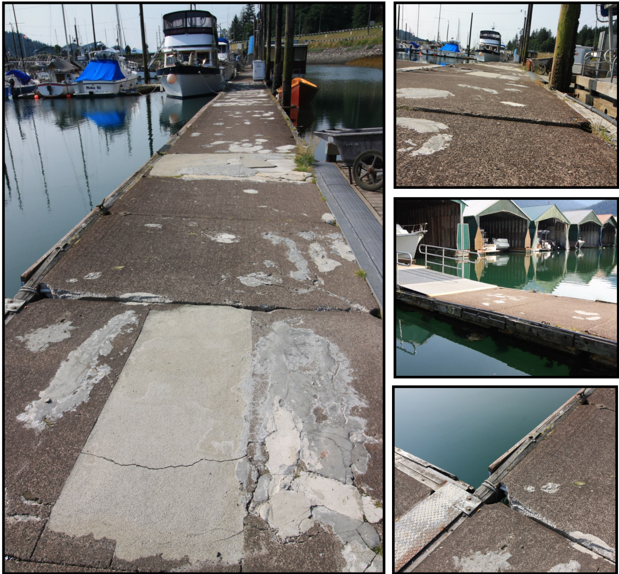
Concrete float wear and uneven float conditions
