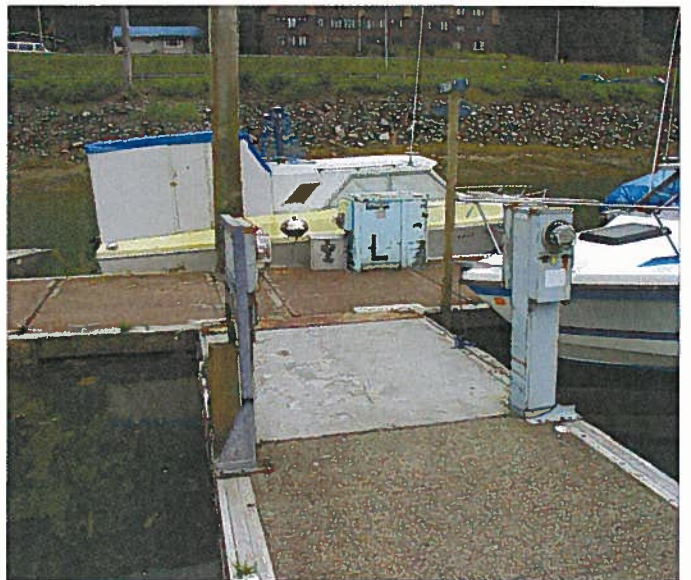
AURORA 100.jpg REPAIRED CONCRETE ON "L" FLOAT
