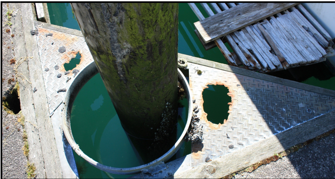
Rusted holes in steel bracing covers
