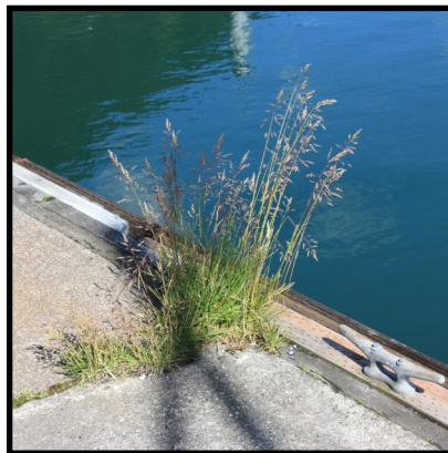
Significant vegetation growth on floats
