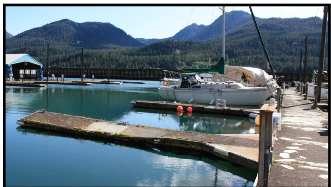
Concrete float wear and uneven float conditions
