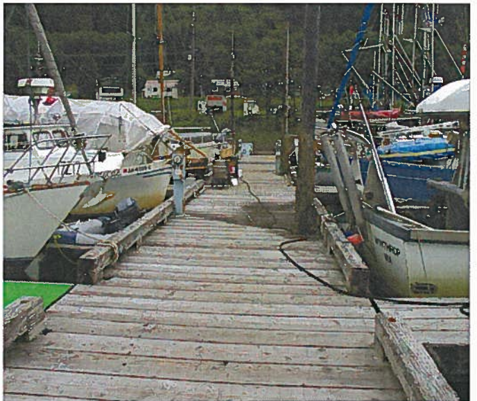
AURORA 076.jpg VIEW EAST DOWN "D" FLOAT
