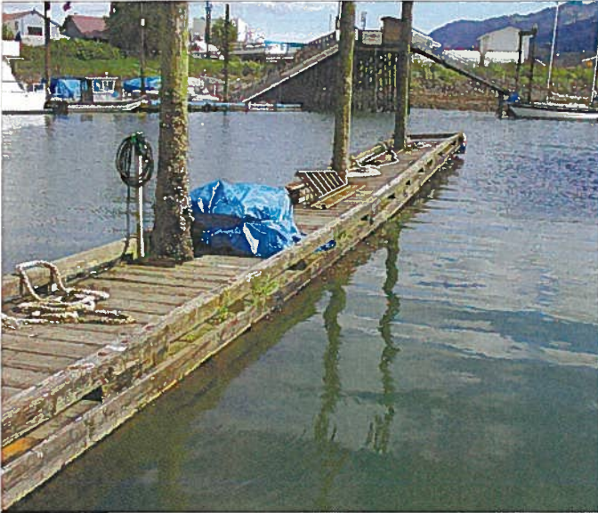
AURORA 067.jpg SAGGING/TWISTED FINGER FLOAT WITH SUBMERGED STRINGERS ON "A" FLOAT
