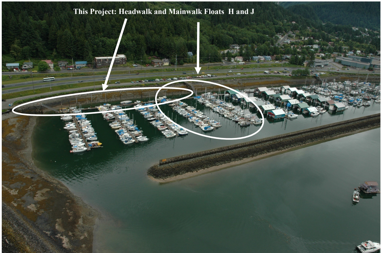
Overall view of Aurora Harbor and project limits
