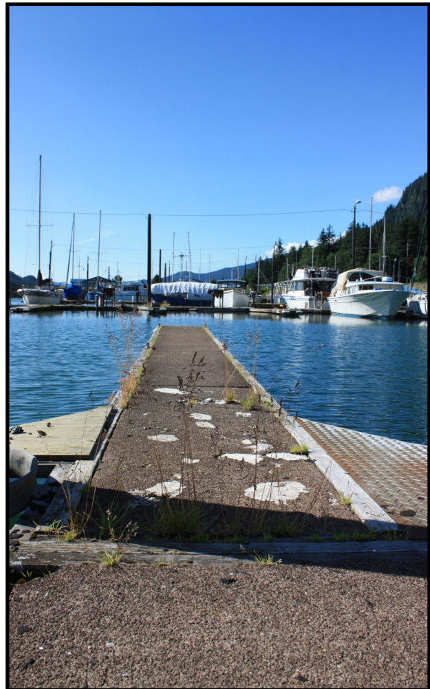
Concrete wear and vegetation growth on floats
