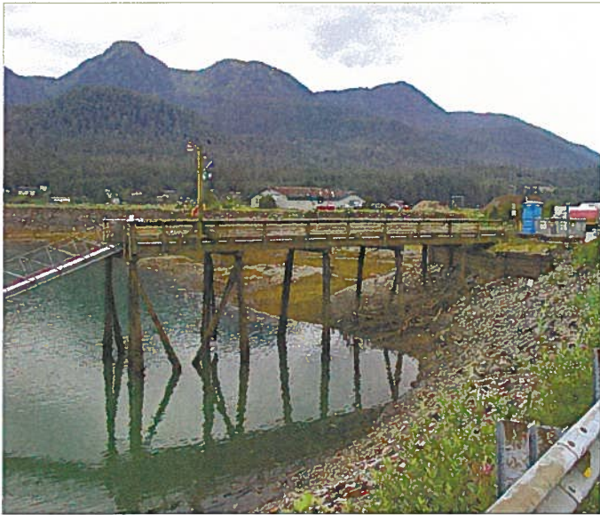
AURORA 055.jpg "N" GANGWAY APPROACH DOCK
