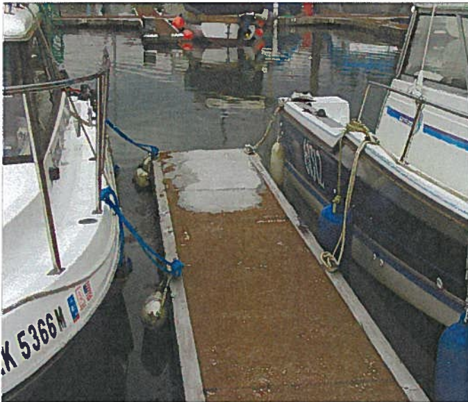
AURORA 097.jpg REPAIRED CONCRETE ON FINGER OFF OF "K" FLOAT
