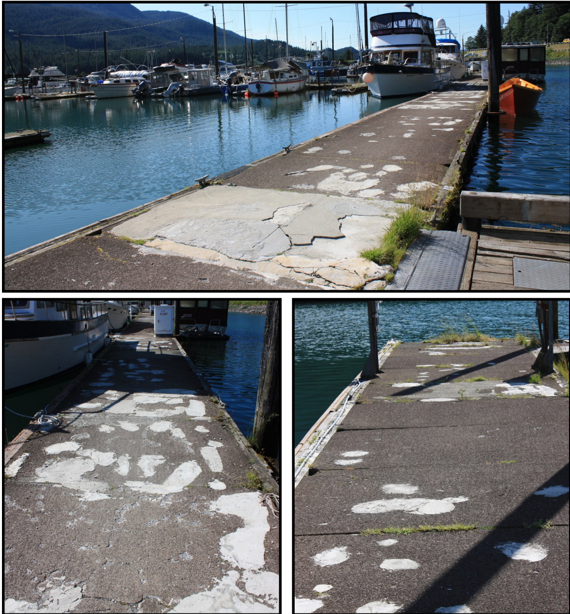
Damaged and patched concrete decking
