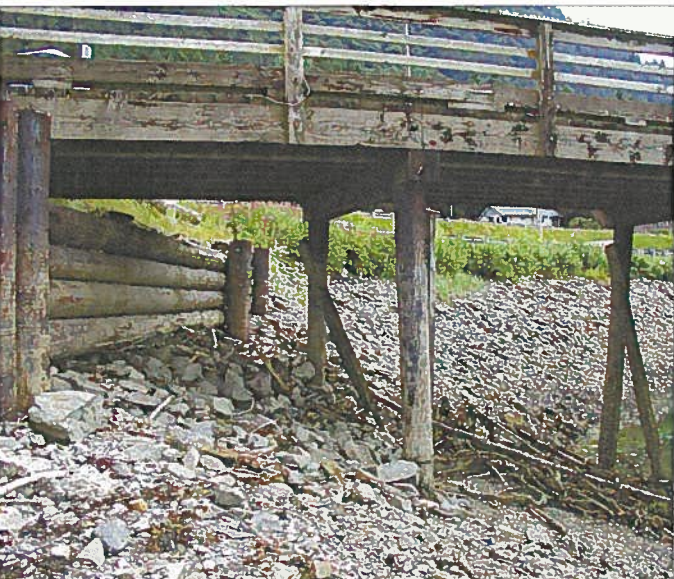
AURORA 065.jpg "N" APPROACH DOCK RETAINING WALL
