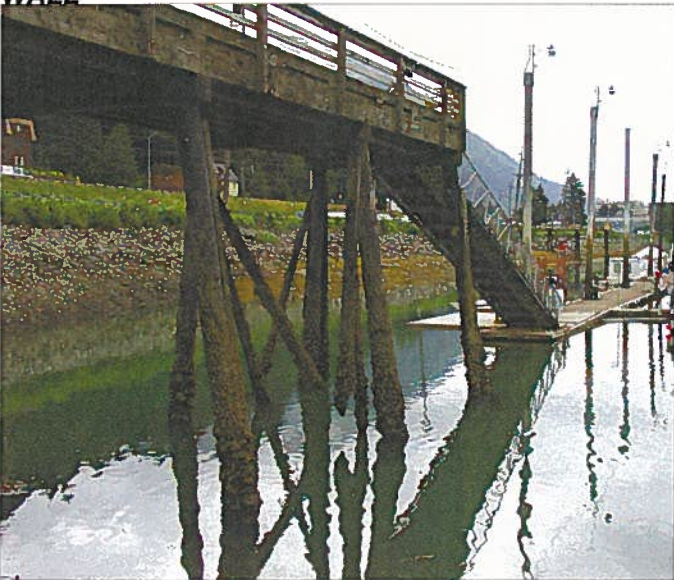
AURORA 063.jpg "N" APPROACH DOCK X-BRACING
