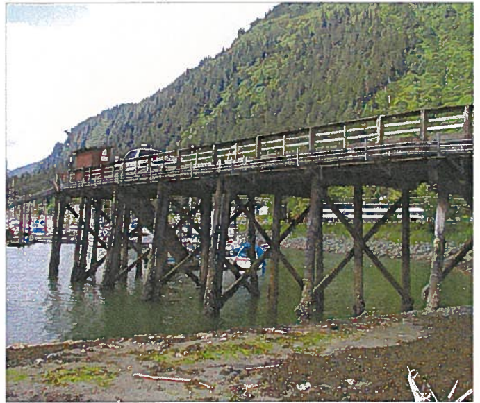
AURORA 002.jpg WEST SIDE OF "A" GANGWAY APPROACH DOCK
