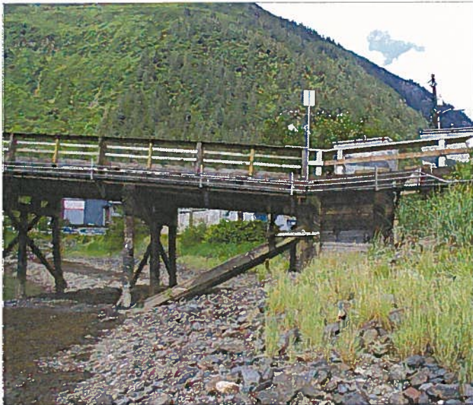
AURORA 003.jpg "A" GANGWAY APPROACH DOCK ABUTMENT
