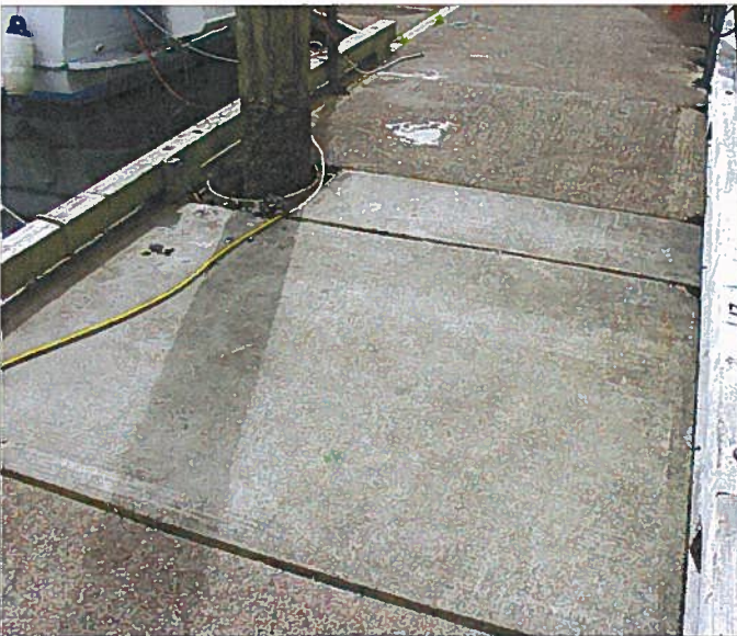
AURORA 087.jpg RESURFACED MAINWALK FLOAT UNIT ON "G" FLOAT
