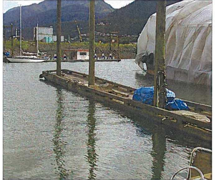
AURORA 068.jpg SAGGING/TWISTED FINGER FLOAT WITH SUBMERGED STRINGERS ON "A" FLOAT
