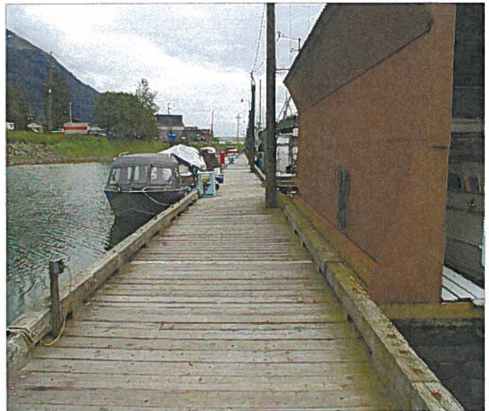
AURORA 026.jpg VIEW DOWN HEADWALK FLOAT FROM "G" FLOAT SOUTH
