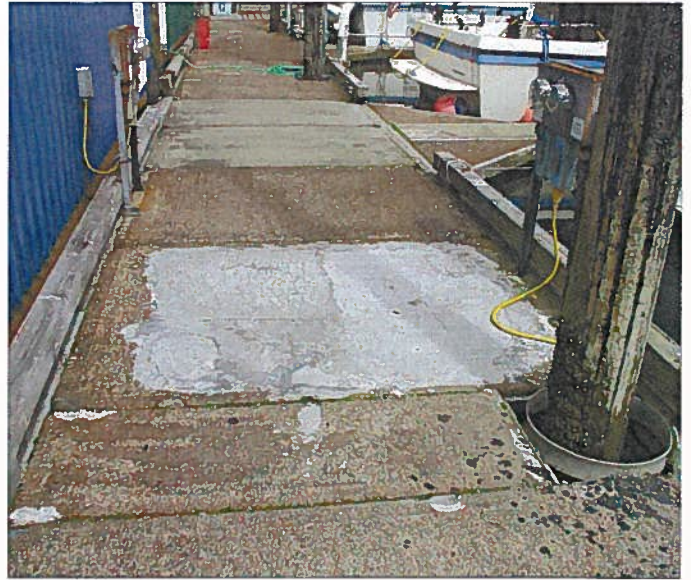
AURORA 086.jpg RESURFACED MAINWALK FLOAT UNIT ON "G" FLOAT
