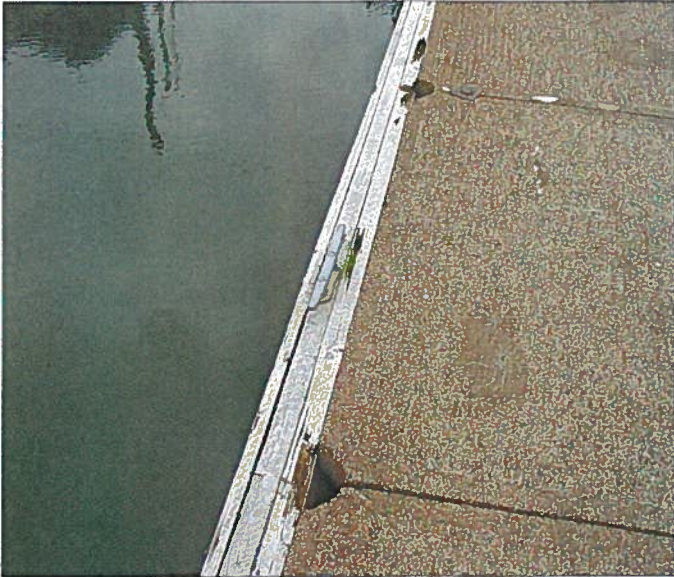
AURORA 049.jpg ROTTEN TIMBER WALERS ON HEADWALK FLOAT BETWEEN "H" AND "J" FLOAT
