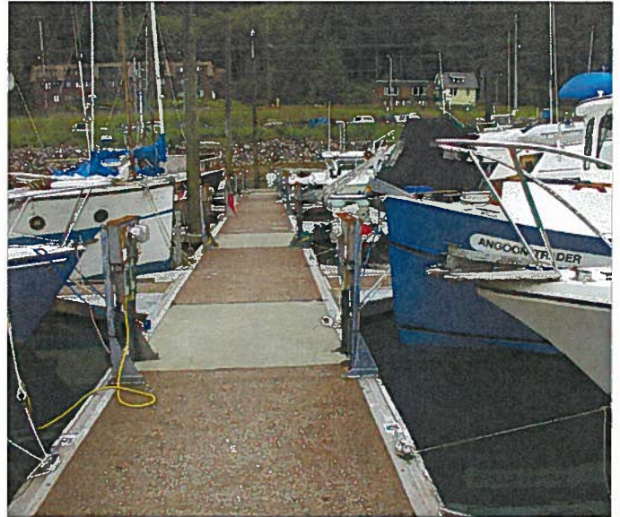
AURORA 092.jpg VIEW EAST ON "J" FLOAT
