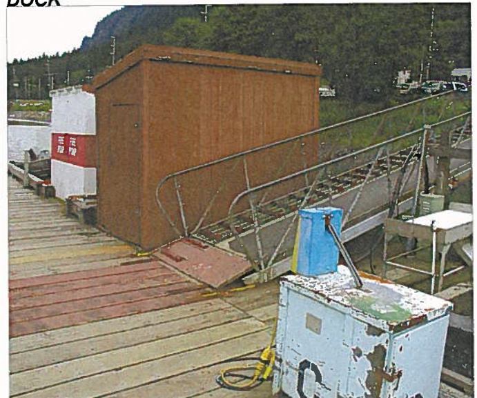
AURORA 012.jpg "C" GANGWAY SKIDS AND TRANSITION TO HEADWALK FLOAT
