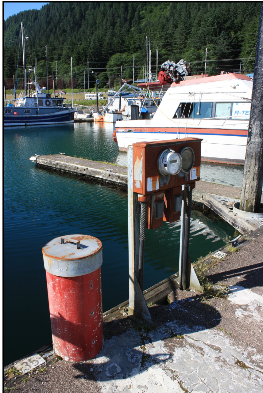
Old and damaged electrical meters
