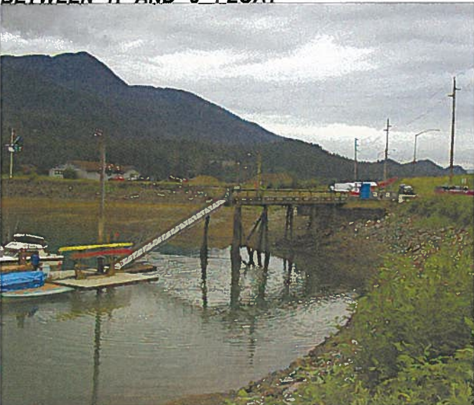
AURORA 053.jpg "N" GANGWAY, APPROACH DOCK AND LANDING FLOAT
