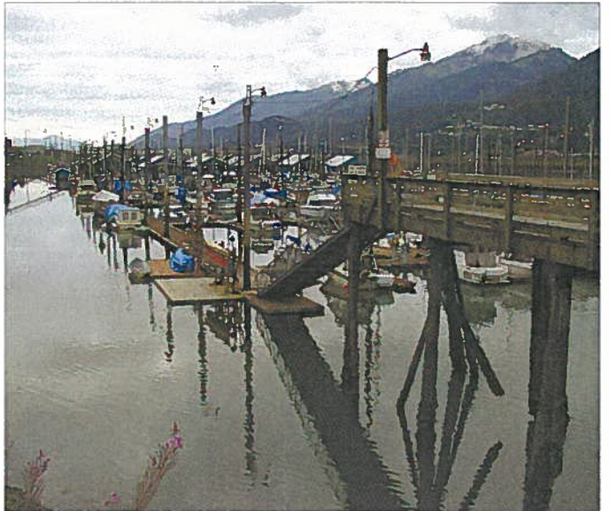
AURORA 060.jpg VIEW SOUTH FROM TOP OF "N" GANGWAY APPROACH DOCK
