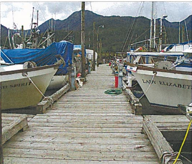
AURORA 077.jpg VIEW WEST DOWN "D" FLOAT
