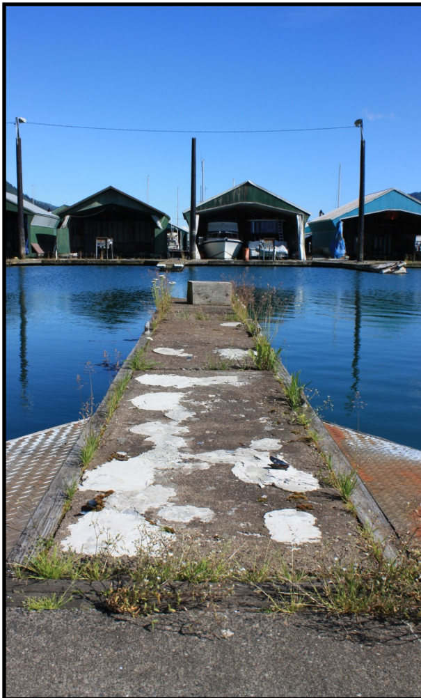
Concrete wear and vegetation growth on floats
