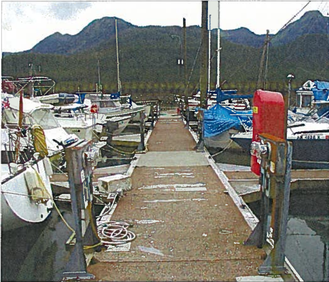
AURORA 091.jpg VIEW WEST DOWN "H" FLOAT SHOWING REPAIRED CONCRETE SURFACE
