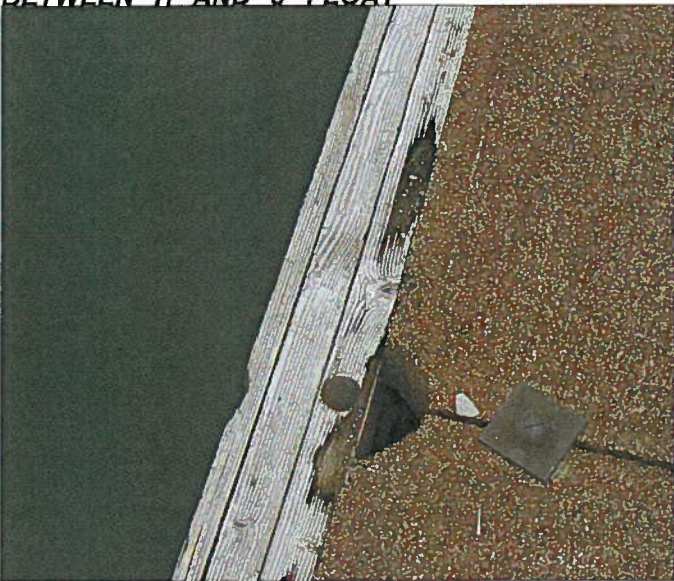
AURORA 051.jpg ROTTEN TIMBER WALERS ON HEADWALK FLOAT BETWEEN "H" AND "J" FLOAT
