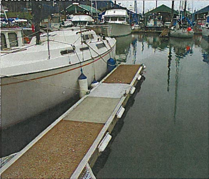
AURORA 093.jpg REPAIRED SURFACE OF "J" FLOAT FINGER
