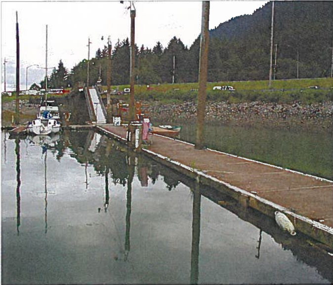
AURORA 043.jpg VIEW NORTH DOWN HEADWALK FLOAT FROM "L" FLOAT
