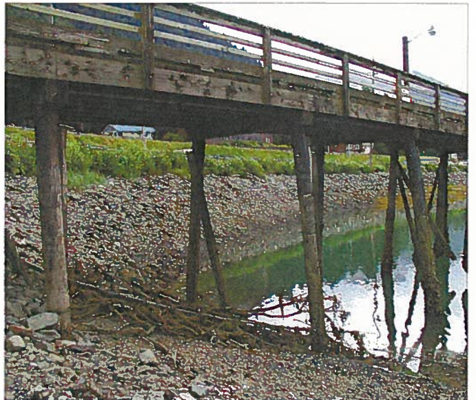
AURORA 064.jpg "N" APPROACH DOCK X-BRACING
