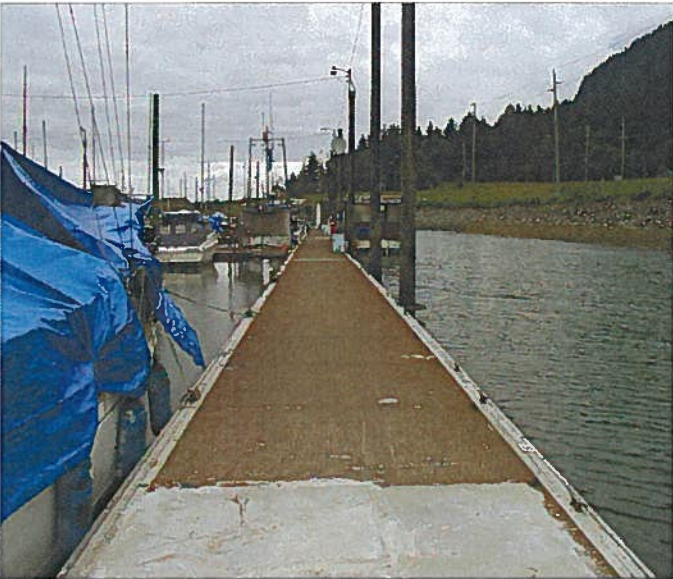
AURORA 039.jpg VIEW NORTH DOWN HEADWALK FLOAT FROM "H" FLOAT
