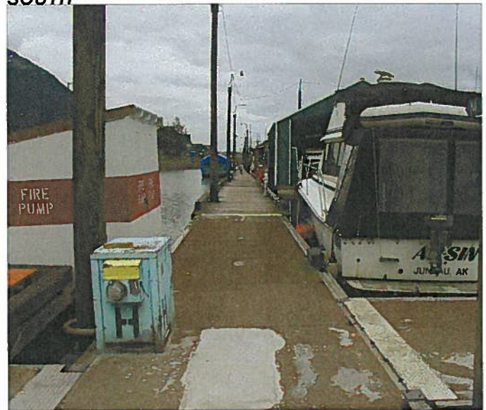
AURORA 028.jpg VIEW SOUTH DOWN HEADWALK FLOAT FROM "H" FLOAT
