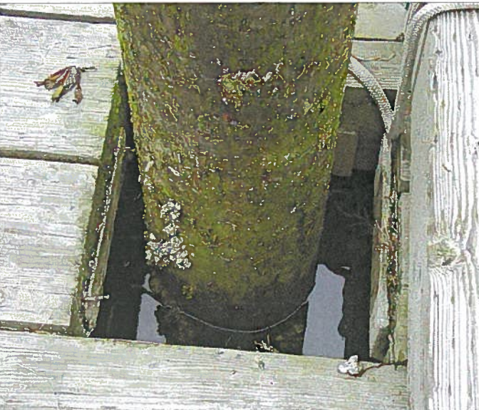
AURORA 071.jpg "C" FLOAT ABRADED PILE AND WORN RUB STRIPS
