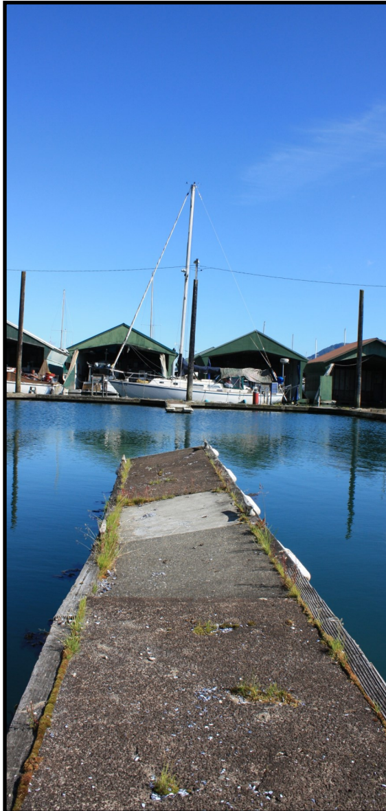
Concrete float wear and uneven float conditions
