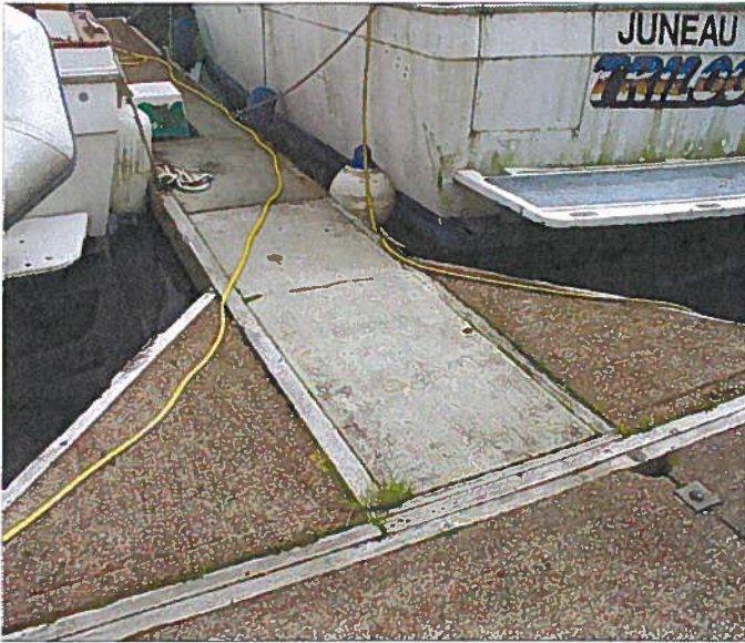
AURORA 085.jpg RESURFACED FINGER ON "G" FLOAT
