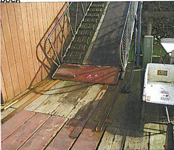
AURORA 021.jpg TRANSITION AND SKID PLATES AT "C" GANGWAY
