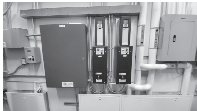
2 EXISTING P-1A/B VFD LOCATION M301 NO SCALE
