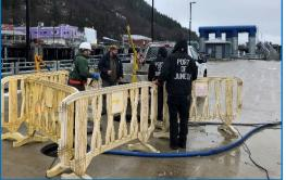
Pumping out the Cruise Ship Pontoon Floats: The Cruise Ship Terminal & Alaska Steamship Docks were placed into service in 2016 & 2017. Although, virtually maintenance-free, one task for the Port maintenance team was to pump out each of the 25 foot by 50 foot cells with accumulated rainwater. There are 56 total cells for the two pontoon floats.
